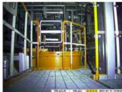
North side manhole
