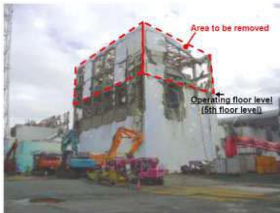
Before debris removal (Southwest surface) Photo taken on September 22, 2011
