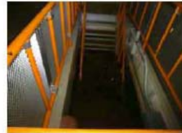
Unit 2 stair case (Northwest)
