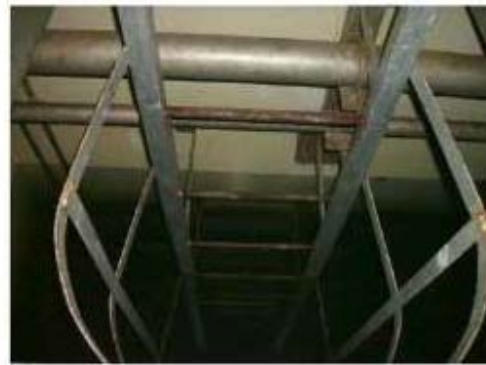
2. North Wall of the Spent Resin Storage Tank Room
