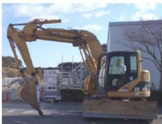
Scraping the road
