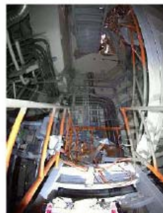
Staircase from 2 nd floor to 3 rd floor
